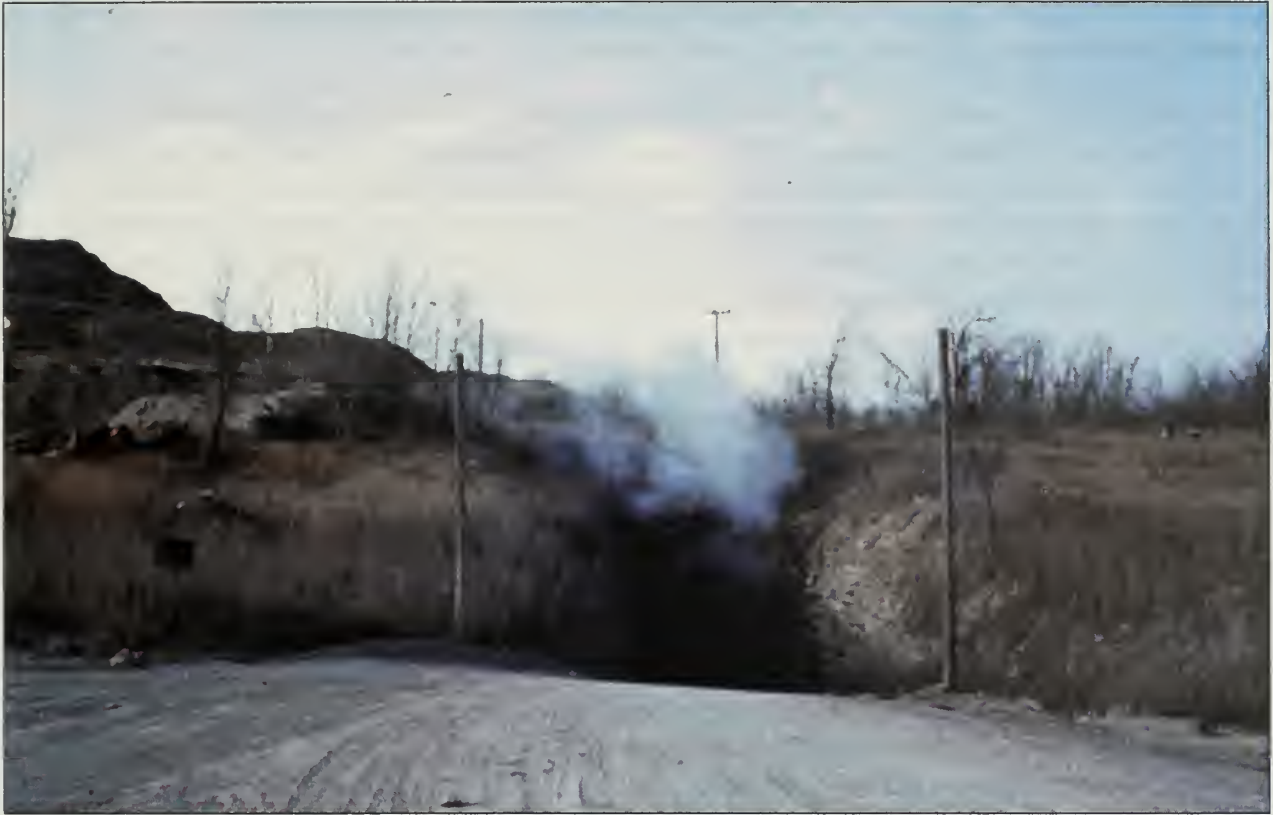
Figure 4 Inclined shaft portal at the Shullsburg mine (circa 1970s). Similar truck access declines replaced vertical shafts during the later years of mining.
